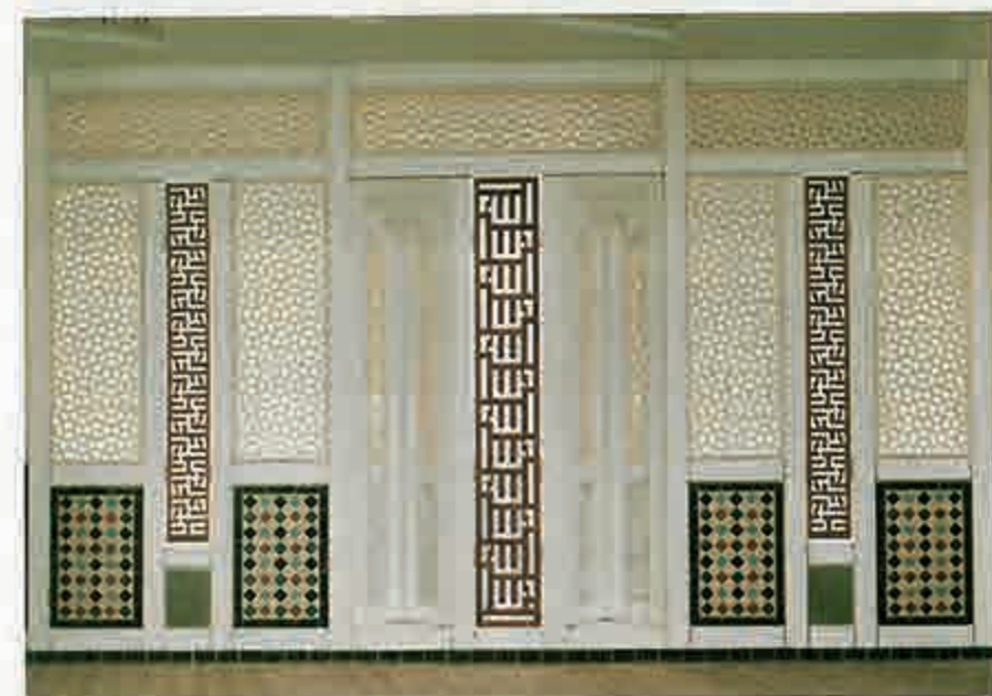
Top left: The bay windows that overhang the deeply recessed west entrance. Top and Top right: The roof garden showing the central fountain connected by radial channels to the four corner pools. Above: Panelling on the west window wall of the Prayer Hall, incorporating marble, tile and plaster lattice panels with vertical teak panels in rectangular calligraphy. The names Allah, Mohammad and Ali are to be read in the light space between the task members. Right: Figure of polished bronze, wood casing. (Hidden and released) height 50cm.
